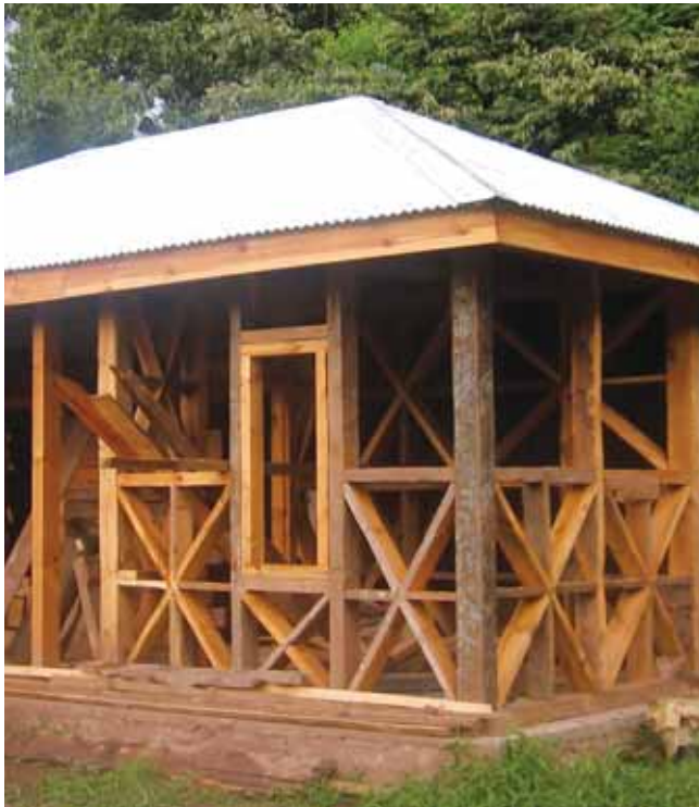
A dhajji design demonstration home with its traditional timber frame construction
