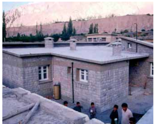
A typical seismic-resistant rural health centre
