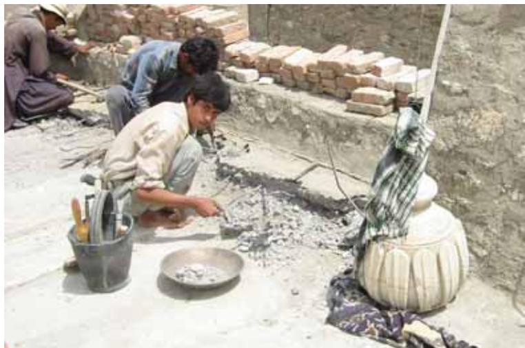
Restoration has involved the removal of reinforced concrete from the mosque roof.
