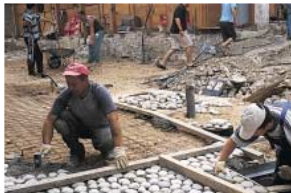
Above: street paving was carried out in the traditional way, with the use of small river stones.
