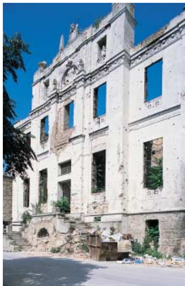
Below: the front façade of the palace in its current condition before the building's imminent restoration.
