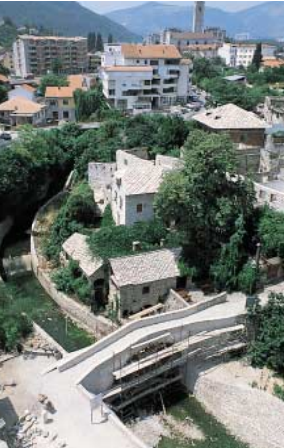
Above: the consolidated Radobolja riverbanks, now part of an improved pedestrian circulation network.
