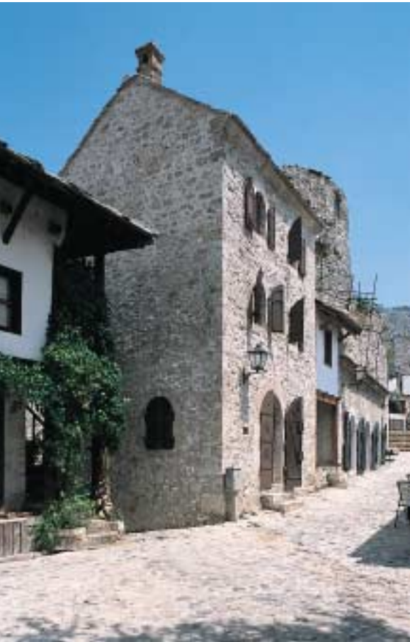
The Ottoman shop tower, located near the western tower of the Old Bridge, was the first rehabilitation project carried out by AKTC/WMF in the Neighbourhood Areas. The use of local limestone rubble, lime mortar and slate for the roof ensure that the original appearance and durability of the building are retained.
