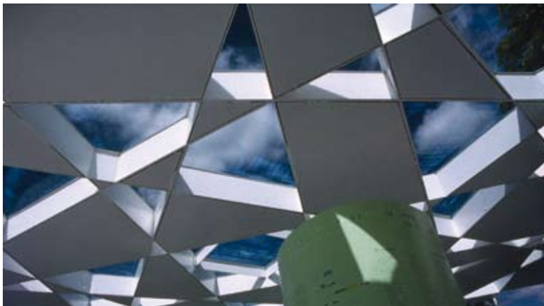
Toyo Ito and Cecil Balmond, Serpentine Pavilion, London 2002. A clear use of a simple algorithm to generate a beautiful structure. This is modified in colour, size and shape to capture its natural green and blue setting in a striking way. (C.Jencks)
