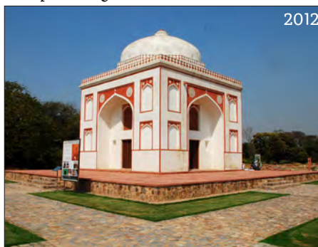
Replastering in lime mortar in 2012
