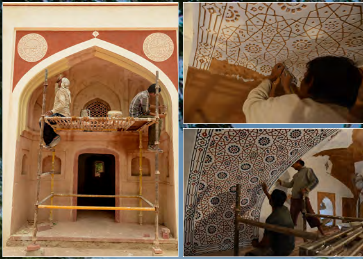
Reviving traditional building craft of Lime Plaster
