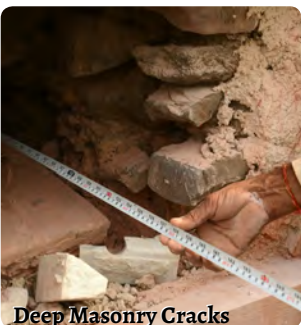
Deep Masonry Cracks
