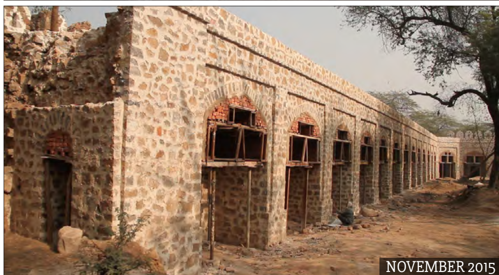
(Above) Collapsed portion of the Serai were carefully stabilized by master craftsmen building with techniques and materials used by the original builders.
