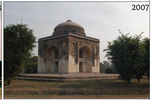
2003 repairs disintegrated, requiring second phase of cement repairs
