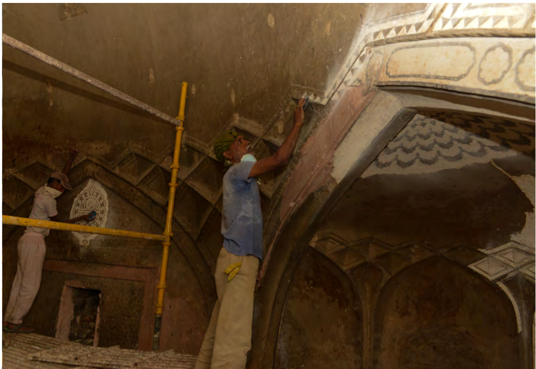
(Above) View of the main tomb chamber before conservation, when it was covered in soot, paint, and limewash; (Below) Main Tomb Chamber during conservation, where the walls and alcoves were cleaned using soft brushes and water.
