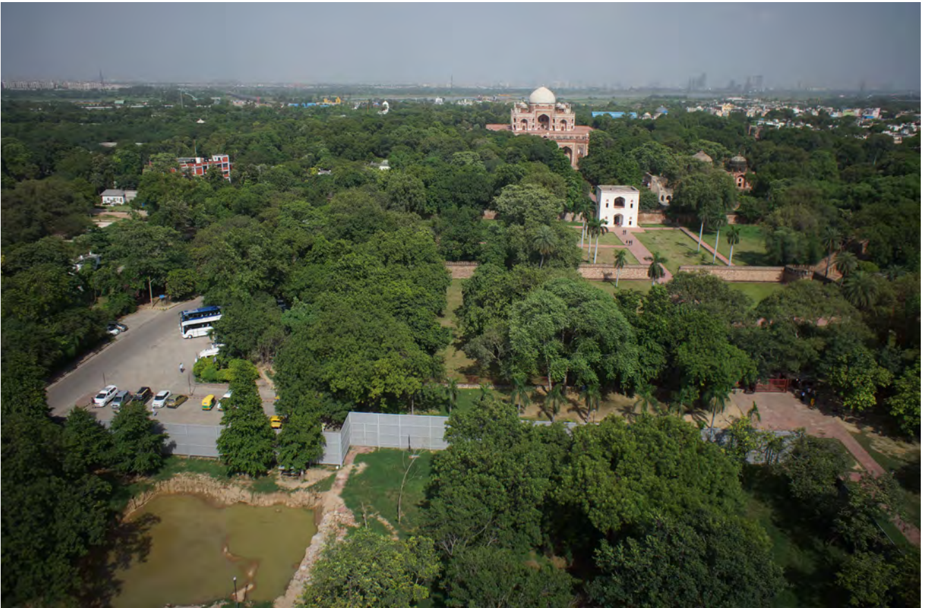
(Above) Construction of the Interpretation Centre commenced in May 2015, after the foundation stone was laid on 7-April 2015
