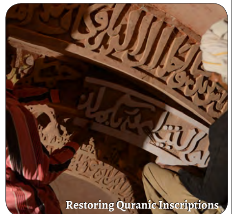
Removal of multiple layers of lead paint
