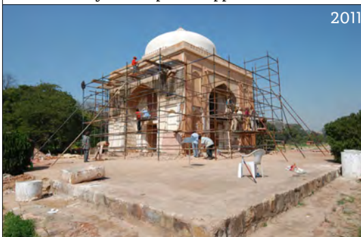
Removal of cement plaster applied in 2003-07
