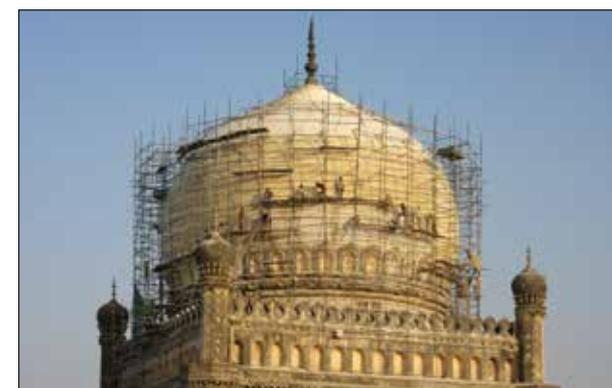
*Conservation works on Sultan Quli Qutb Shah's Tomb (top) required replacing cement plaster with traditional lime plaster; and re-building of its garden enclosure wall after its original foundations were excavated (centre); Over 60 masons worked tirelessly to apply a traditional lime plaster layer on the dome of Muhammad Quli Qutb Shah (bottom).*
