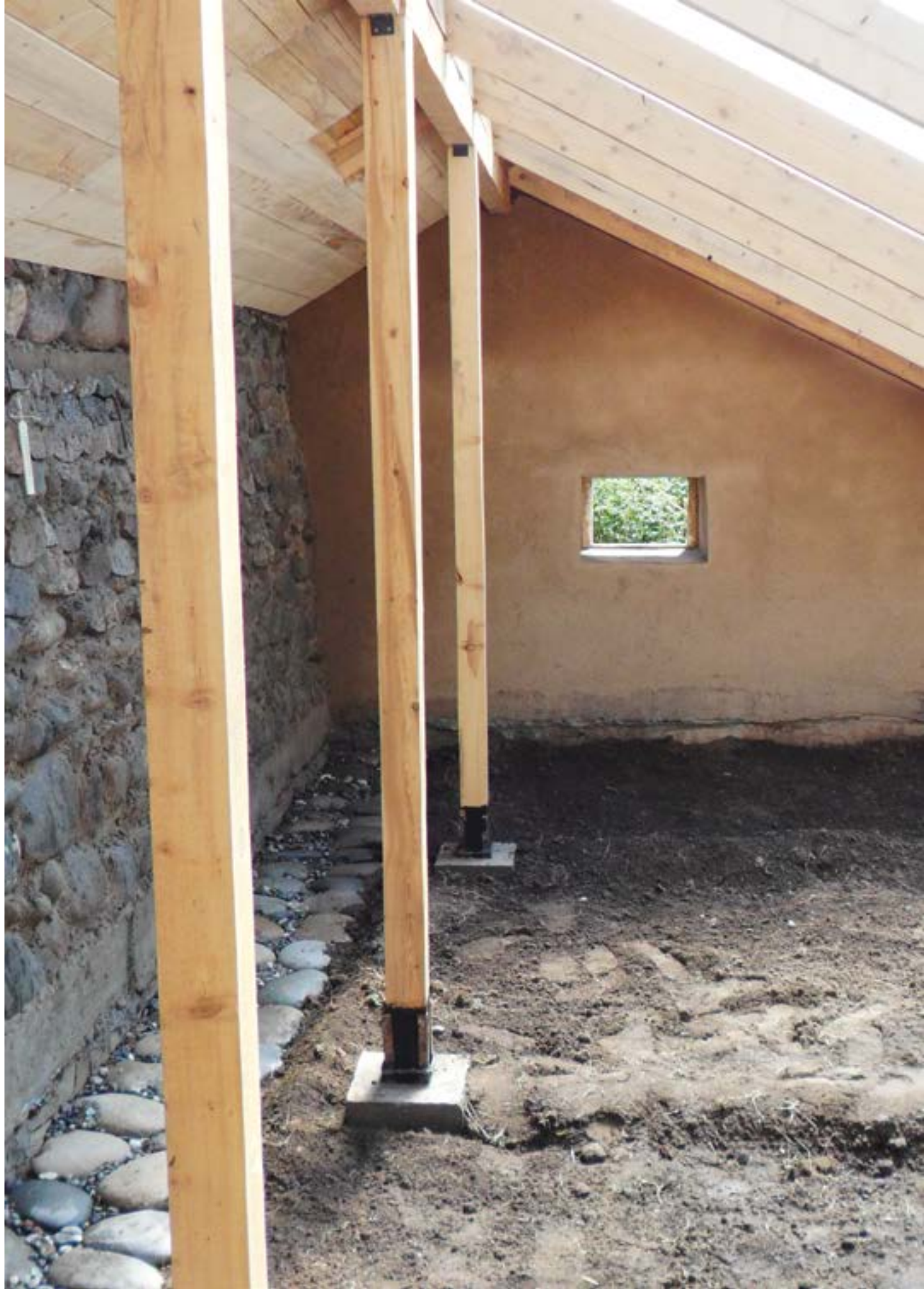
The Chinese-style solar greenhouses are perfectly adapted to the climatic conditions of Naryn Oblast. This greenhouse can maintain an above-zero temperature without any additional heating even when the outside temperature is as low as -20^{\circ}\text{C} , thanks to the stone walls which absorb and keep solar energy.
