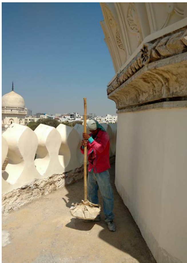
The cement from the terrace was replaced with traditional lime concrete
