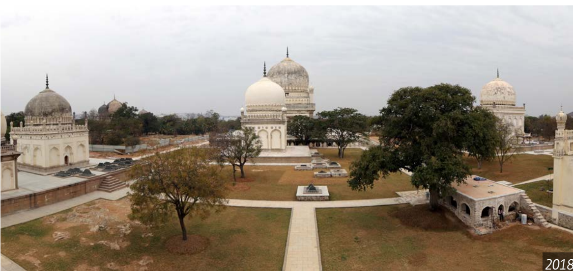
Conservation of the monuments is being coupled with sensitive landscaping their immediate surroundings; creating a historically appropriate setting. Landscape development included the removal of modern interventions, restoration of original earth levels, laying of stone pathways and plinth protection around the monuments.
