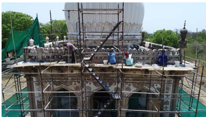
(Right) Parapet of the Hakim's mausoleum during conservation
