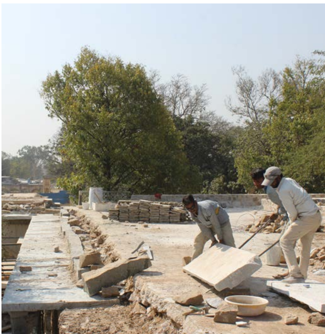
Stone eaves installed on the facade of serai
