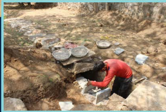
Channelization of rain water from adjoining areas into the Baoli
