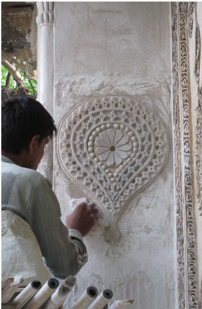
(Left) Restoration of lime stucco details on the facade; (Top Right) Installation of granite stone edging around the 'wazu'tank; (Bottom Right) Installation of hand chiseled dressed stone steps
