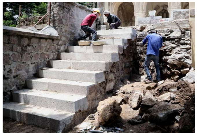
(Left) Restoration of lime stucco details on the facade; (Top Right) Installation of granite stone edging around the 'wazu'tank; (Bottom Right) Installation of hand chiseled dressed stone steps
