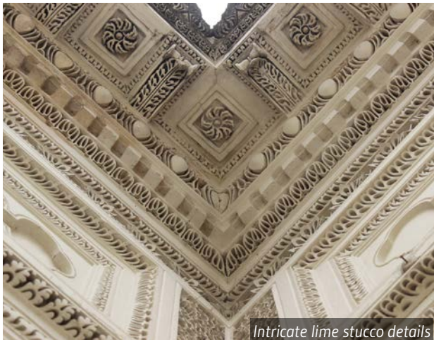
Intricate lime stucco details
