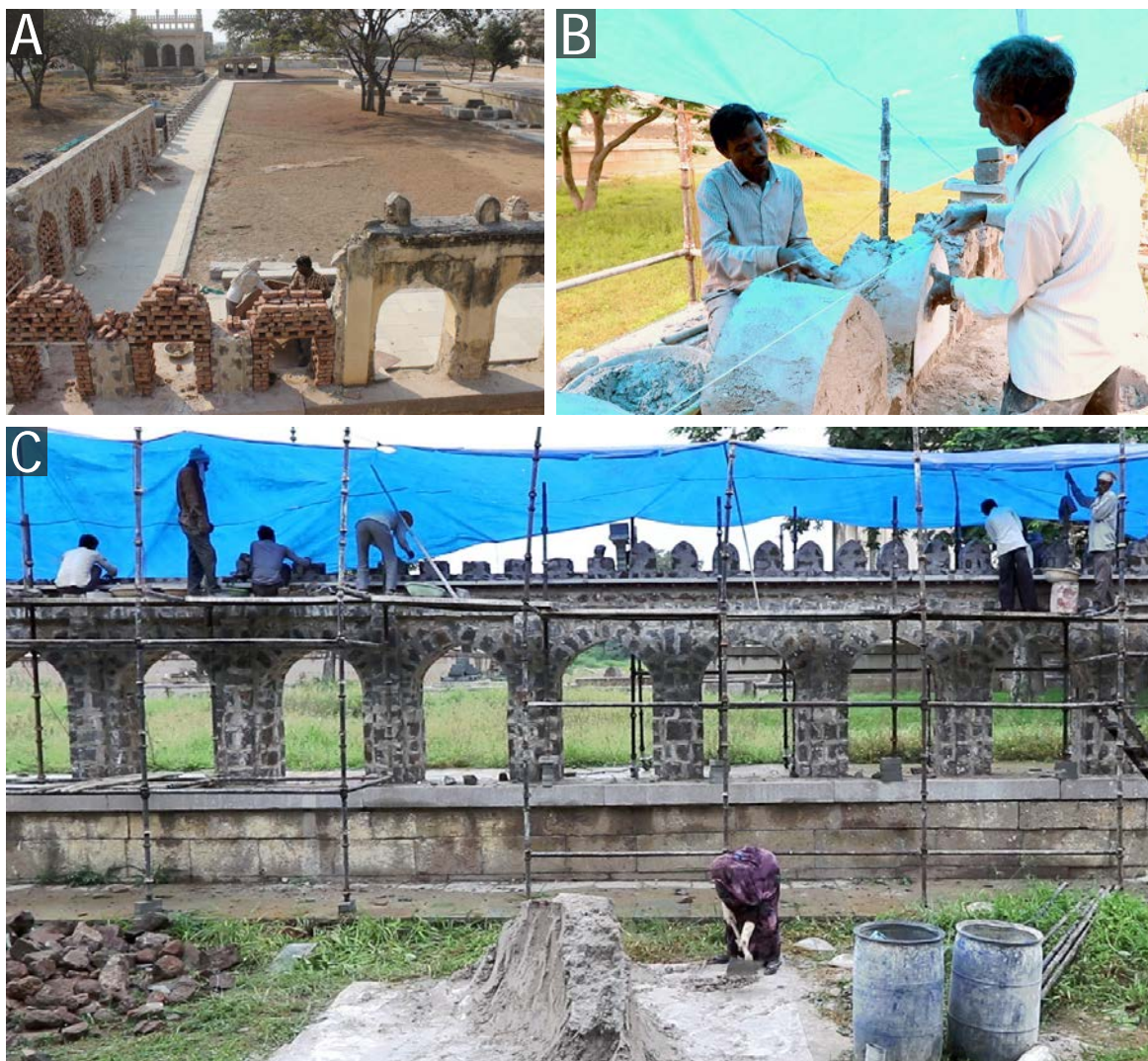
A: Honeycomb brick shuttering for construction of arches; B: Plastering of masonry battlements above reconstructed arcade; C: Reconstruction of battlements in stone masonry
