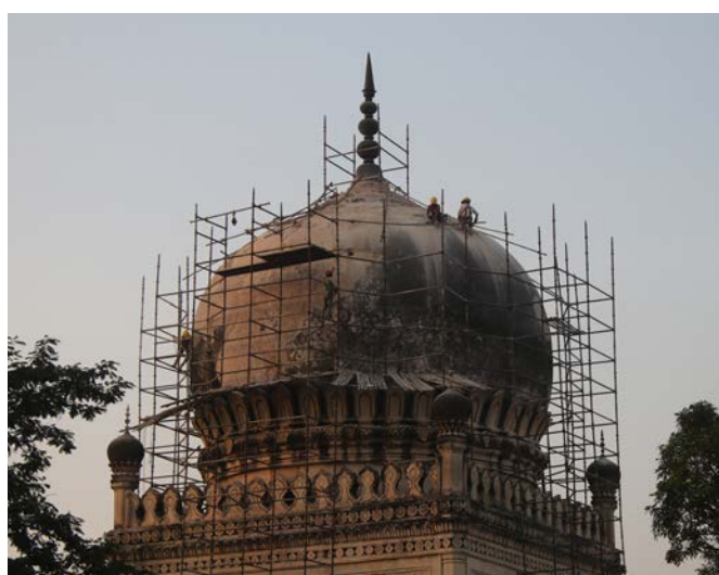
Removal of 6 inch thick cement layer
