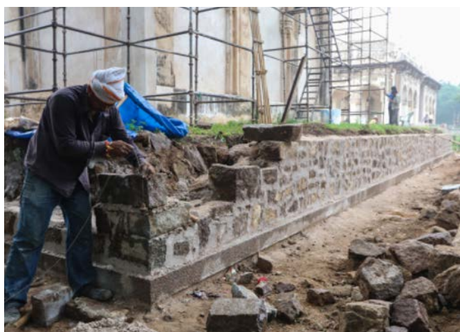
The plinth wall at Commander's mausoleum was bulging due to water ingress, was hence dismantled and followed by reconstruction with stone and lime mortar and installation of hand-chiseled stone coping
