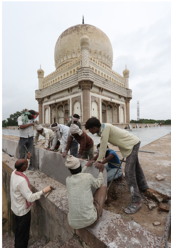
125 hand chiseled dressed stone blocks with profile matching the archival evidence were installed after removal of the 20 th century metal railing
