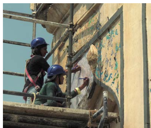
(Top) Outline of the missing detail on the facade were restored; (Middle) Missing stone elements added to the external blind arches on the facade; (Bottom) Physical documentation of existing tiles by architects
