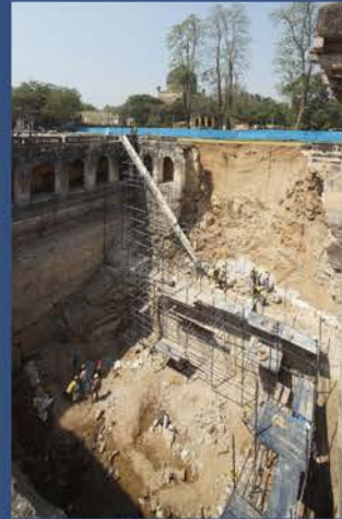
Reconstruction of masonry arches above western wall at Badi Baoli
