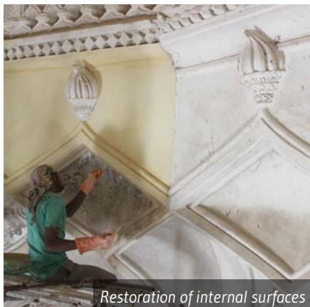
Removal of damaged and loose plaster layers
