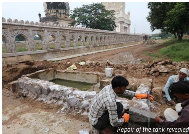
Steps installed for access
