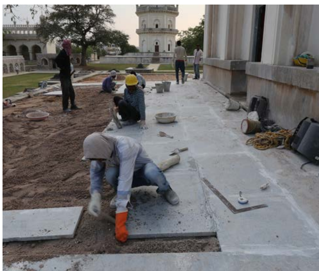
Removal of cement concrete from the plinth to halt further deterioration Laying of stone slabs on a layer of lime mortar to replace the cement
