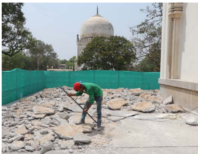
Removal of cement concrete from the plinth to halt further deterioration Laying of stone slabs on a layer of lime mortar to replace the cement
