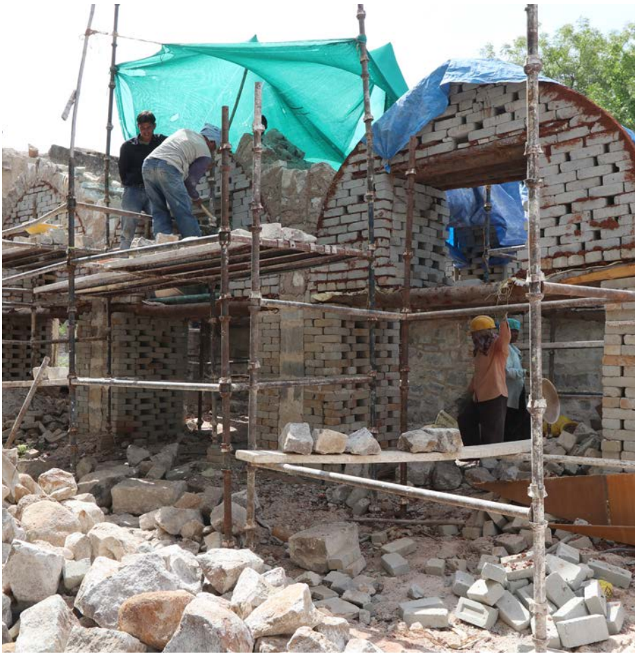
(Left) Reconstruction of arcade using traditional honeycomb shuttering (Top right) Installation of stone beams on the reconstructed arcade's roof; (Bottom right) Ramming of the lime concrete laid on top of the stone beams
