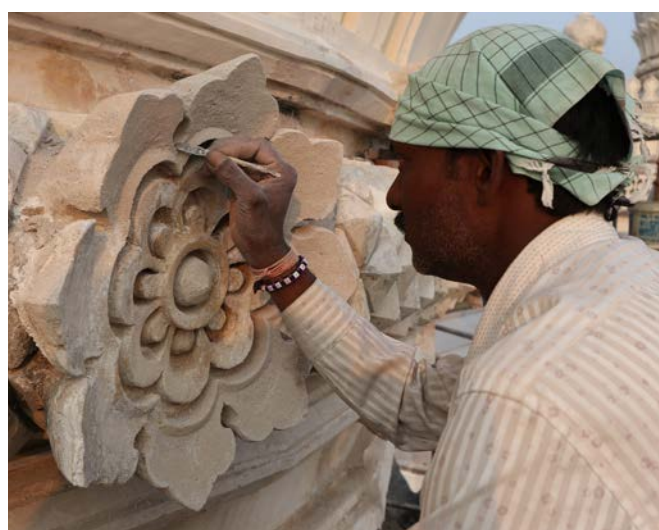
Restoration of ornamental detail
