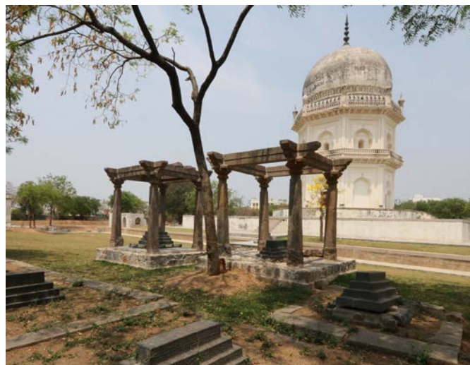
The collapsed pieces were reinstated in their original position
