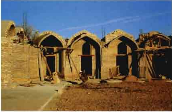
The arcade of the Ruhabad madrasa under reconstruction by the State Institute of Restoration.
