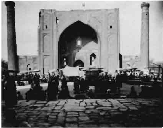
A turn-of-the-century photograph of Ulugh Beg's madrasa, completed circa 1420, shows the thirty-five-metre-high central pishtaq without the tile mosaic decoration restored in recent decades.
