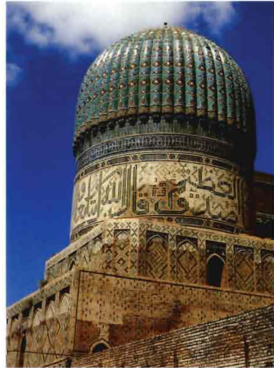
A detail of the reconstructed ribbed dome of the Bibi Khanum mosque.
