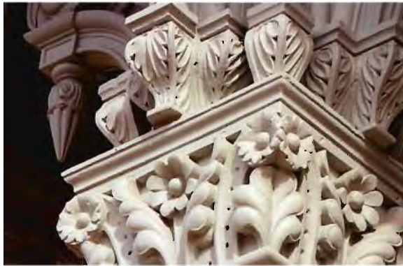
Detail of a sculpted plaster capital on the ground floor veranda.
