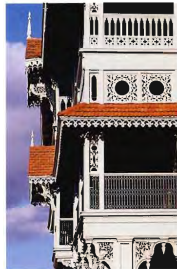
Views of the front balcony, wood joinery, and ornament, before (above) and after (below) restoration.
