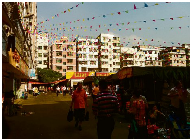
FIG. 3: The urban village of Baishizhou, Nanshan District, Shenzhen. The villagers' buildings are so close that it is possible to reach out a window and shake hands with one's neighbor. This is an image of the area's vibrant central public space, which serves as a basketball court during the day and a market at night.
