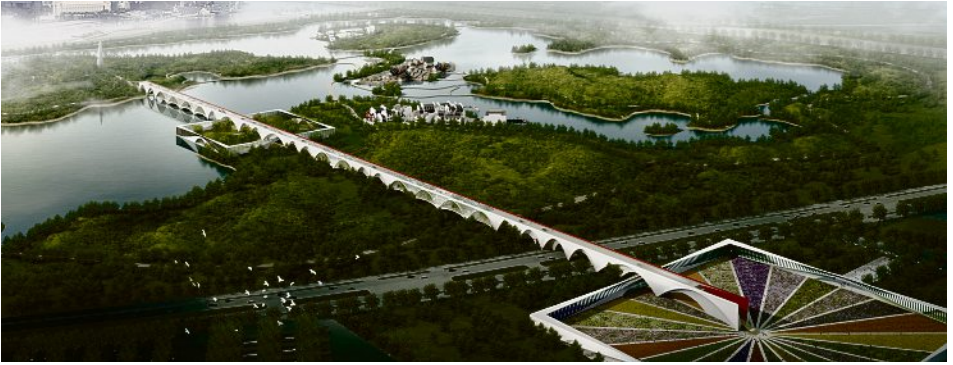
FIG. 5: Design proposal by Serie Architects for five greenhouses for the Xi'an Horticultural Expo: Aerial perspective. The wall is reimagined as a one-kilometer-long, multilevel footbridge that cuts across the horticultural park and the Shibo Avenue motorway.
