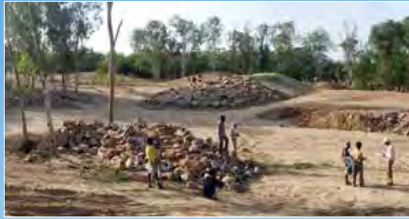
2. Boulders and rocks carefully collected from various sites across Delhi and surrounding regions and carefully arranged on the mounds to recreate a 'kohi' or ridge-like appearance.
