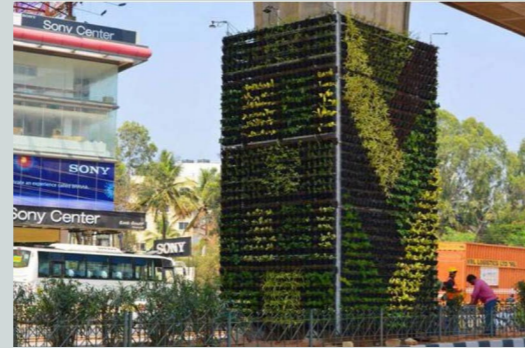
Figure 83: Image showing Vertical Gardens in Bengaluru
