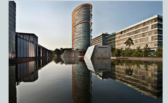
Figure 77: Image showing blue roofs in Walter Bos Complex, Apeldoorn
