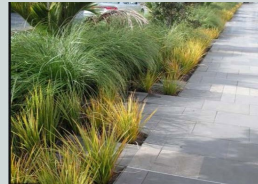
Figure 75: Image showing bioswale in Jellicoe Street, Auckland, New Zealand
