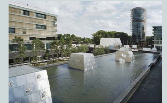
Figure 78: Image showing blue roofs in Walter Bos Complex, Apeldoorn
