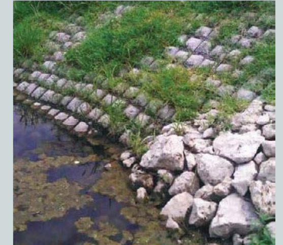
Figure 98: Image showing slope stabilization in French Broad river bank in Tennessee, USA
