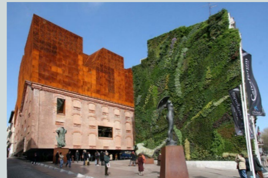
Figure 84: Image showing Vertical gardens in Caixa Forum plaza, Madrid
