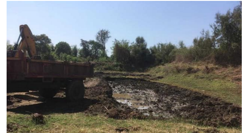
Figure 60: Construction along Vasai Creek
