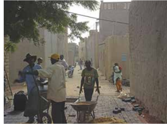
Above and opposite: In Mopti, restoration of the Mosque of Komoguel was linked to a water supply and sanitation programme aimed to improve environmental health in the neighbouring area (above). As part of this programme, the AKDN operated a manufacturing facility to produce street-paving blocks made of recycled plastic bags and sand (opposite).
