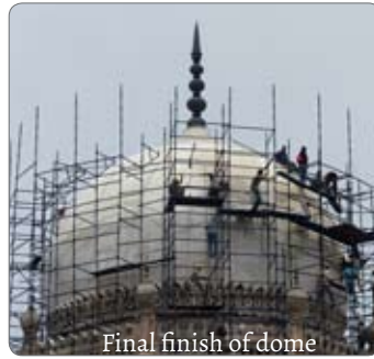
Final finish of dome
