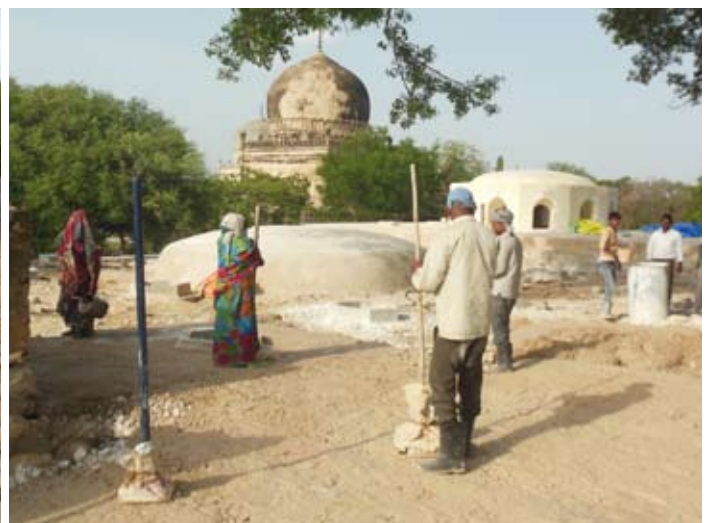
(Left) Removal of cement from the roof; (Right) Laying of traditional lime concrete on the roof after dismantling of cement
