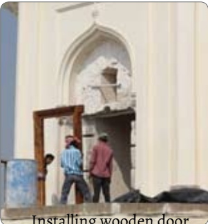
Installing wooden door
