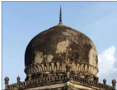
Present-day view where the tiles seem to have been plastered over
