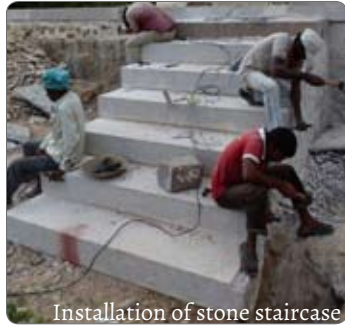
Installation of stone staircase
