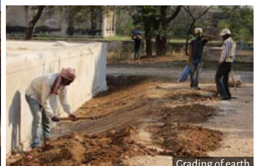
Grading of earth
