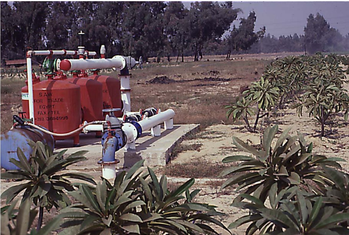
IRRIGATION METHODS CAN RANGE FROM THIS PUMP/FILTRATION STATION AT THE DESERT PLANT NURSERY OF AL- AZHAR PARK IN CAIRO TO WATERING PLANTS BY HAND FROM ROPE-AND-BUCKET WELLS.
